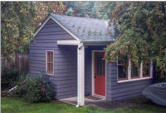
A Detached ADU (Photo by Lauren Flemister, City of Tacoma)
