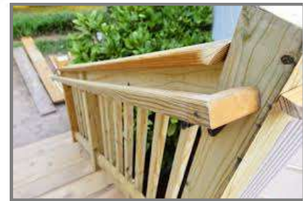
Stairs with guardrail and a handrail
