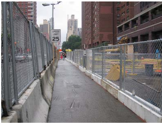
Temporary asphalt sidewalk
