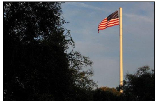
Wireless Tower Camouflaged as Flagpole
